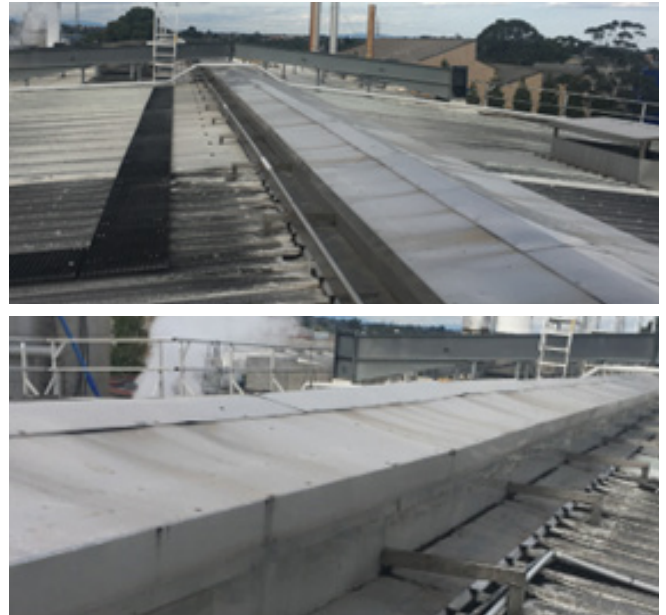
Figure 3: Ridge Vent – Post Sealing
