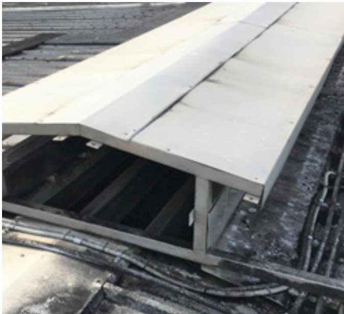
Figure 2: Ridge Vent – Pre-sealing
