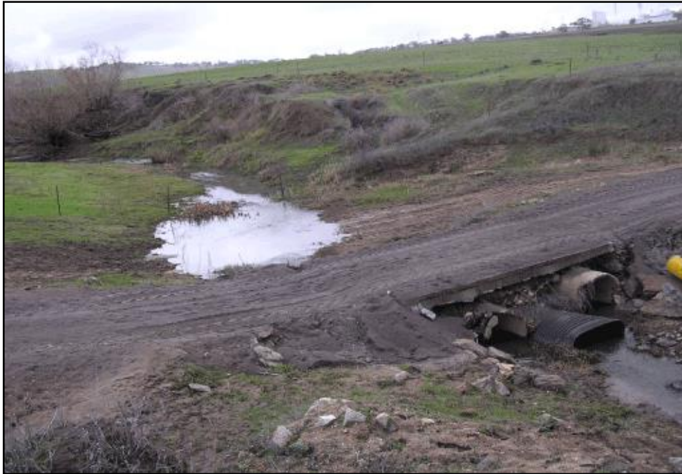
Figure 14: Surface water monitoring point number 5
