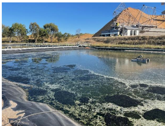
Cooling Pond 3B
