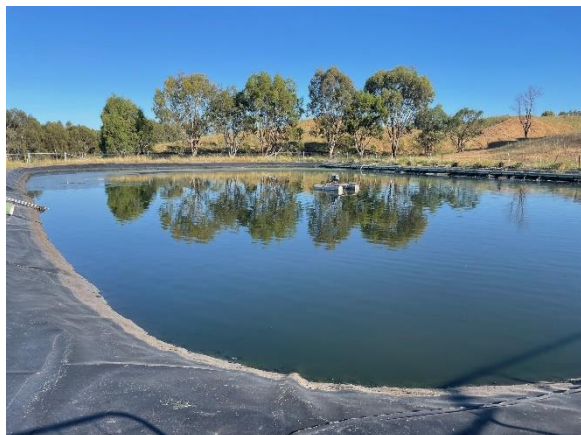
Cooling Pond 3A
