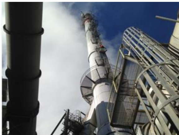
EPA 1 - Main Stack 1
