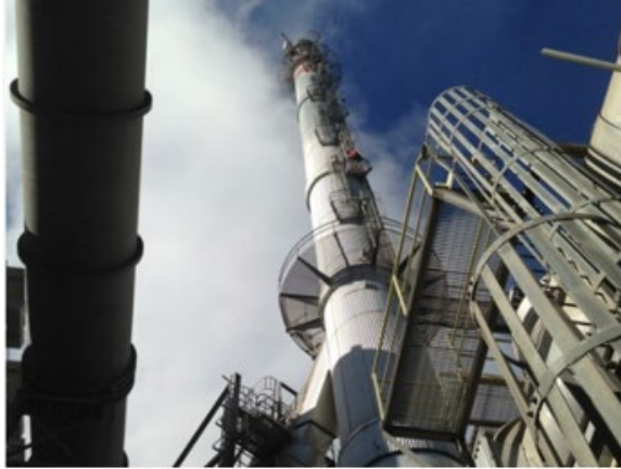
EPA 1 - Main Stack 1
