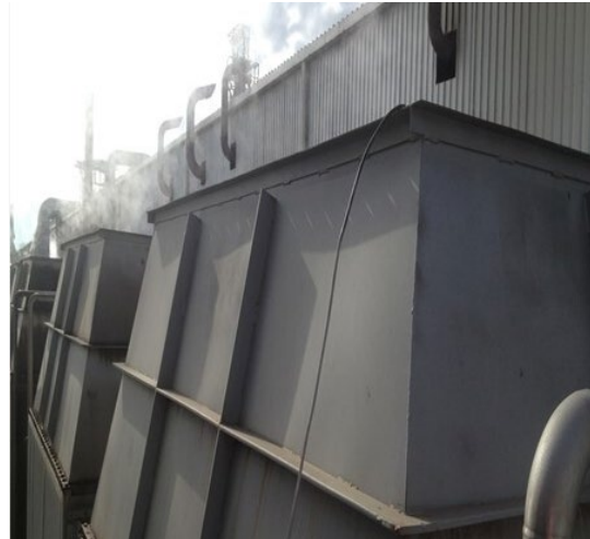
Vacuum Pump 10 (Paper Machine Hood Vent Exhaust)
