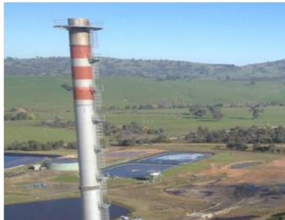
EPA 22 - Main Stack 2
