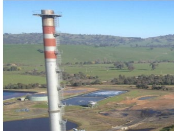
EPA 22 – Main Stack 2
