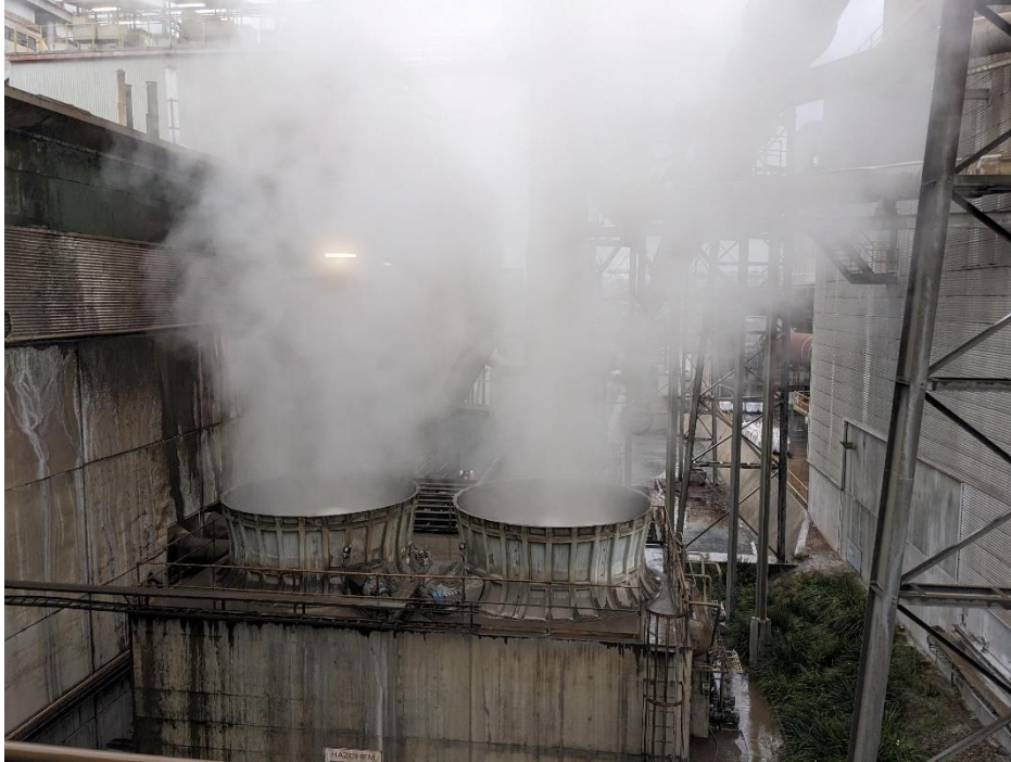
Evaporation area adjacent the site control room
