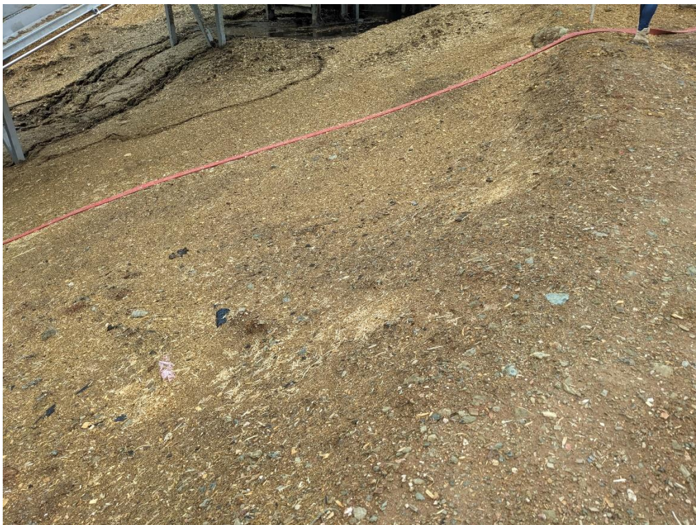
Woodchip residue providing effective erosion control within the Wood Yard
