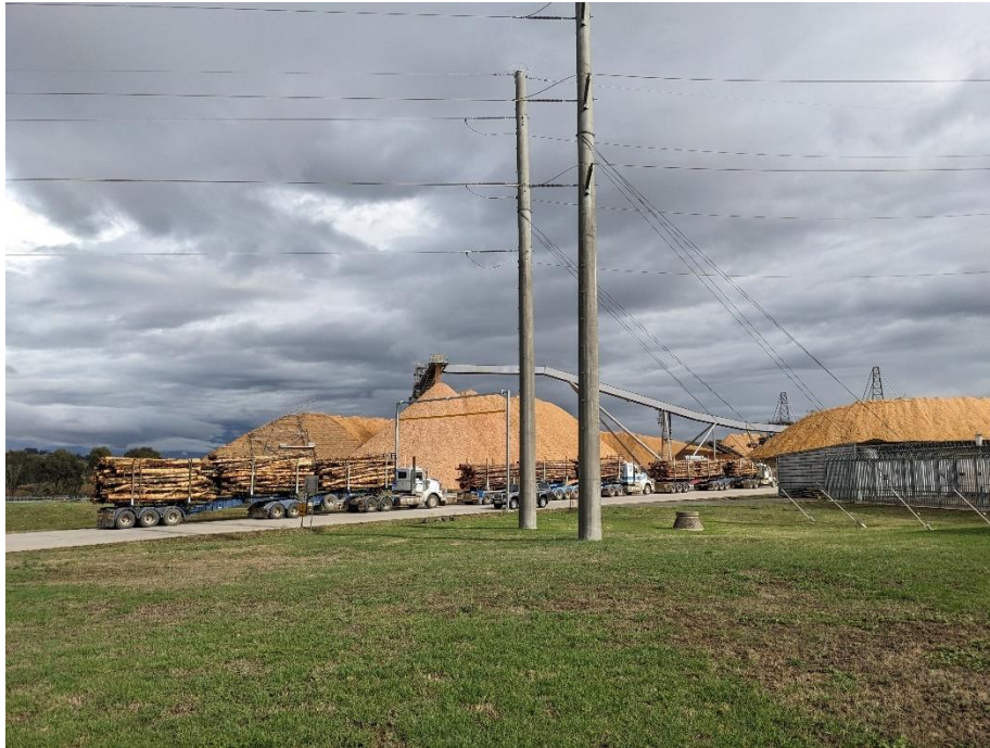
New stacker reclaimer in operation
