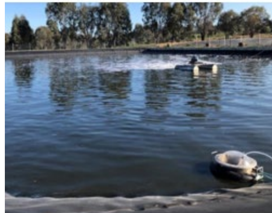
Cooling Pond 3B
