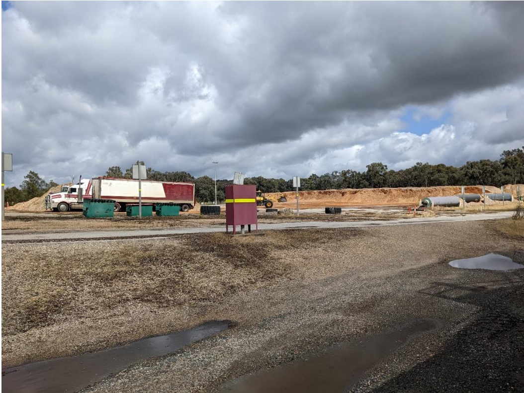
Woodchip yard – all logs on site have been chipped and are being removed for use at Visy Tumut
