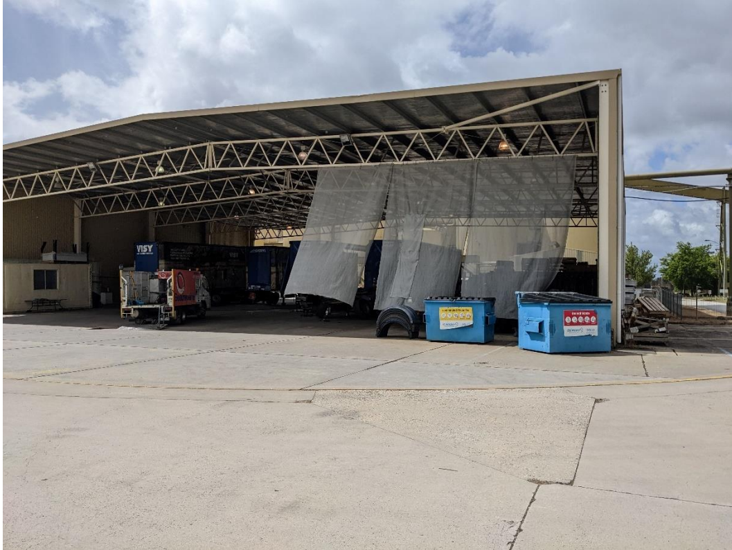
Visy Logistics utilising the workshop facility for basic truck body maintenance
