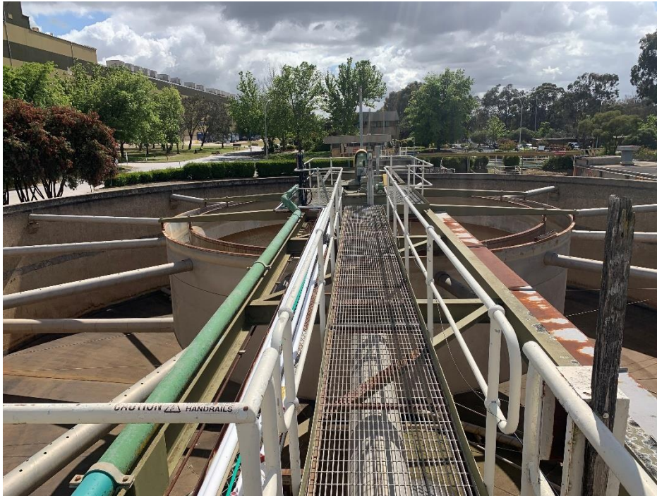
Wastewater treatment infrastructure not in use
